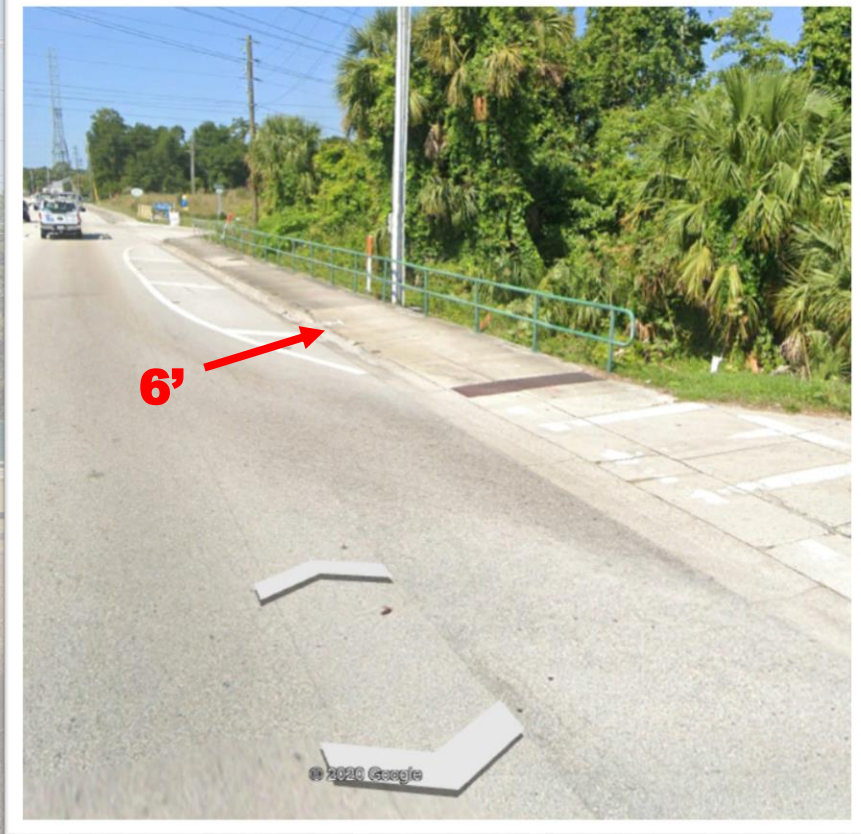
Bridge on Ronald Reagan Blvd between Bay Meadow Drive and Longwood Lake Mary Road
