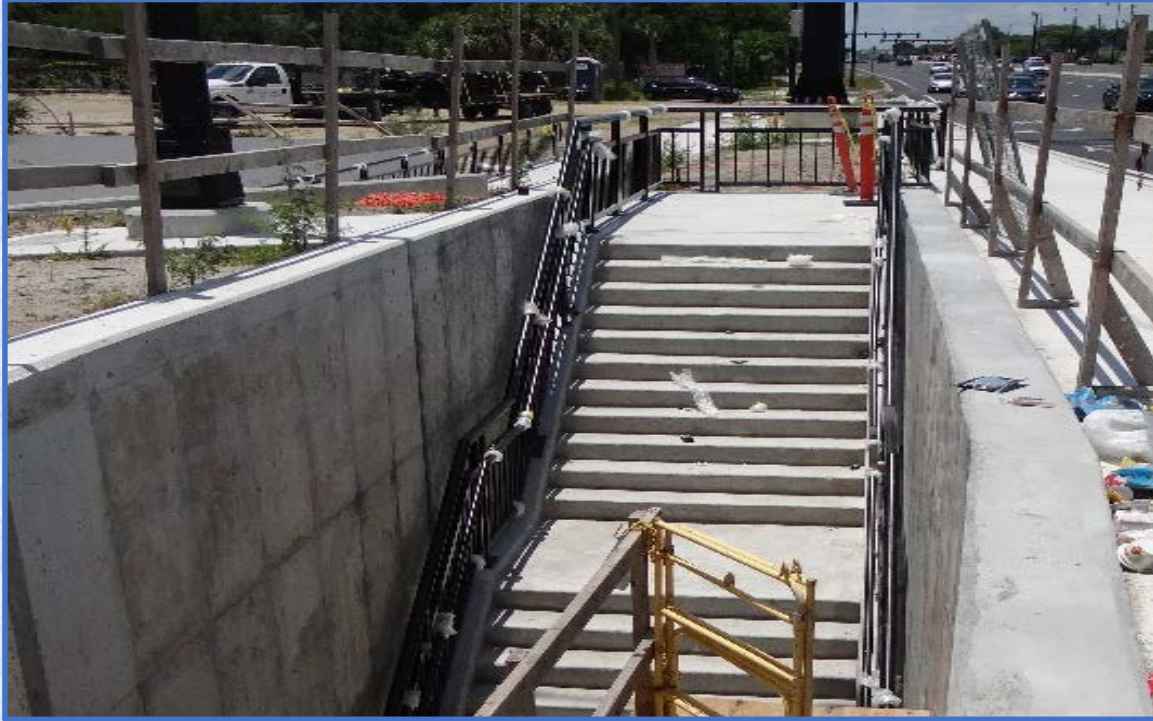
Stairway Access in Addition to Approach Ramps
